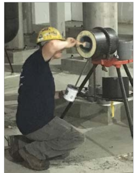
COOL-FIT is easily joined using cement and a flat brush. Pictured is Mike Sharp, Leadman for M. Davis & Sons, Inc., the Delaware-based contractor most heavily involved with the COOL-FIT installation at Dogfish Head.
